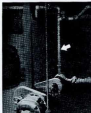
Heating cable applied to pipe line carrying molasses
